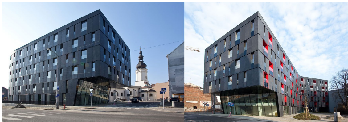
Figure 3 – Apartment house Ostravska brana (source: archiweb.cz)
